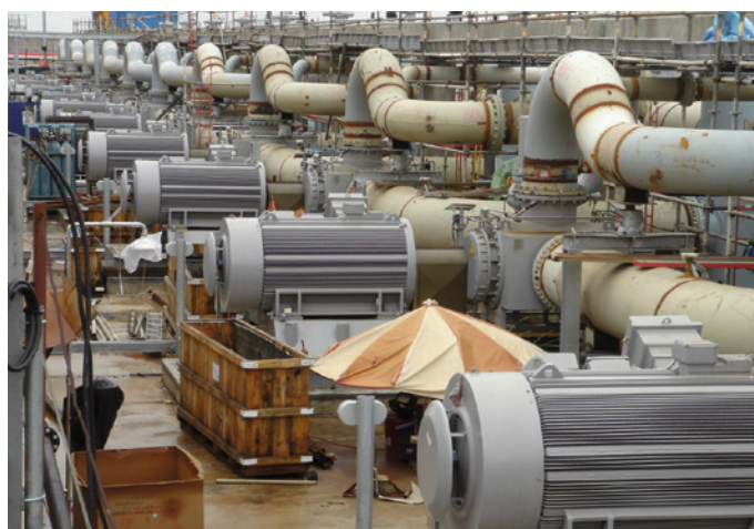
L2- and L5-series pumps for unloading oils from trucks and railcars have only one sealing to the atmosphere while the L4-Series can offer an interchangeable liner. These pumps are self-priming and have run dry and solids capabilities.
